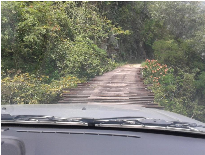
Figure 2. Wooden bridges at some sections of the road to the target.
